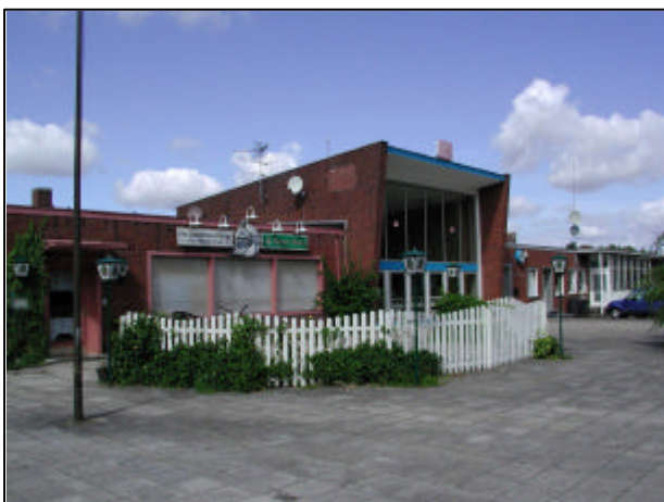
The Espelkamp station building before its renovation.
