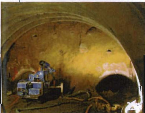
Above: Excavating the Langallerie tunnel Right: Fig 1 - M2 alignment with tunnels
