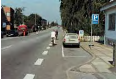
The parking bays here are too narrow. A car door is 0.9 m wide.
