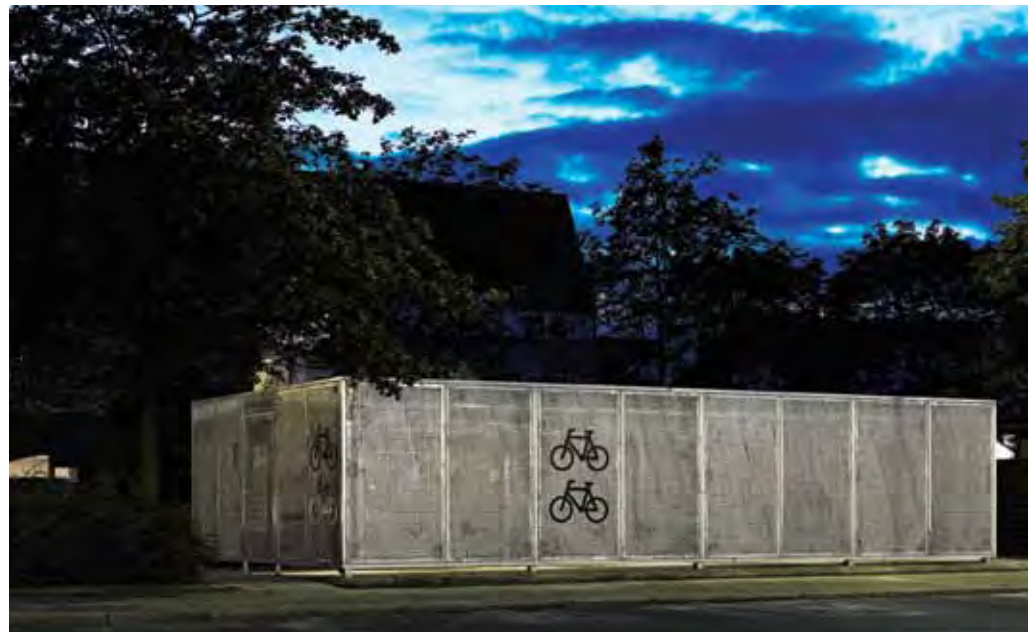
Lockable bicycle parking facility, Randers. Solar cells on the roof power LED lighting in the facility.
