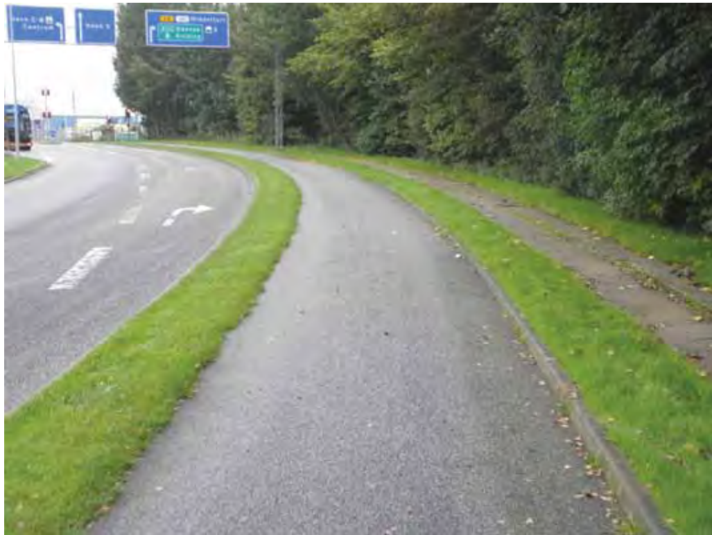
A cycle track with a verge is excellent on highways and on road sections without side roads
