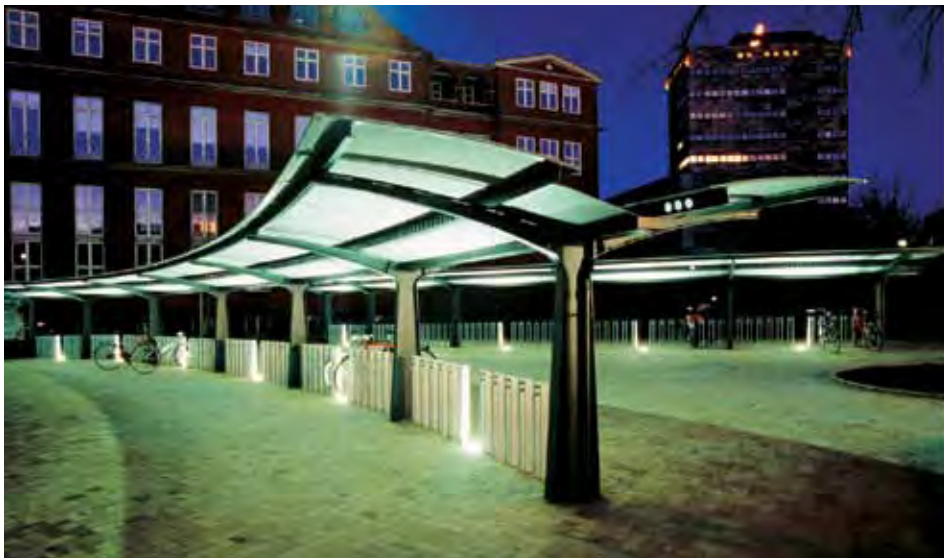
Covered bicycle parking facility at Kinopladsen, Odense, at night.
