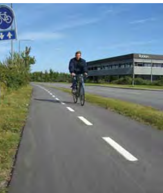
Two-way cycle track along Kragholmen in Frederikshavn. The solution works well as there are no side roads.
