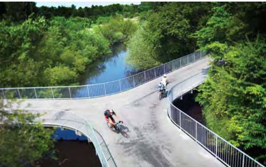
Well designed bridge.
