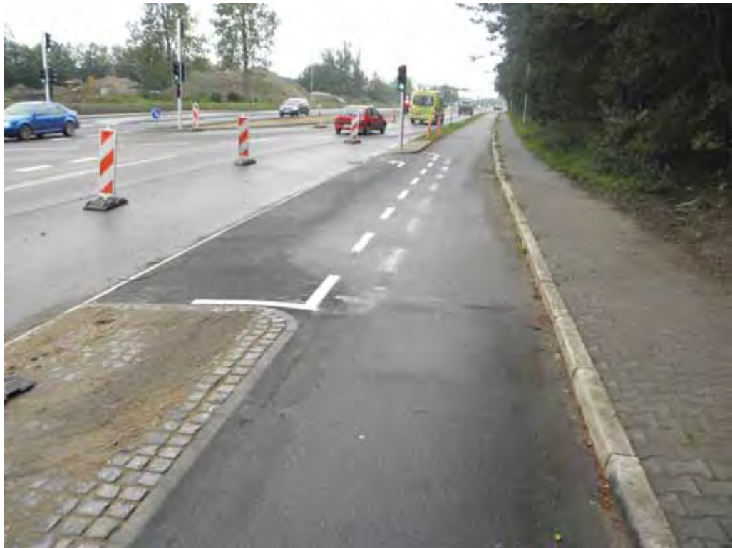
Cyclists going straight ahead pass the traffic signal, while cyclists turning left have their own signalized lane.
