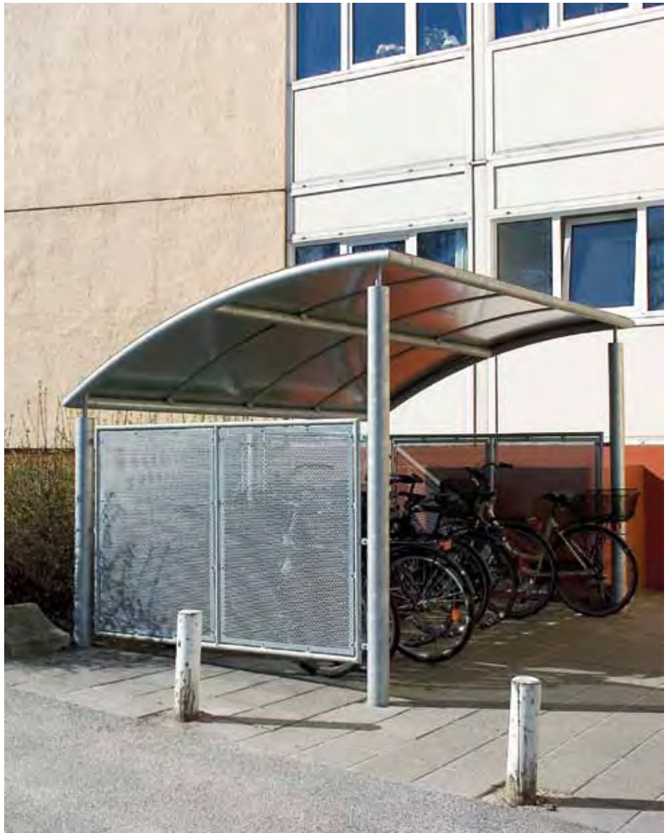
Covered bicycle parking facility at block of flats
