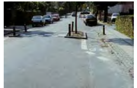
Cycle gaps, manhole covers, debris, and parked vehicles are an unfortunate combination.
