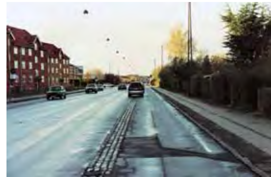
Segregation of road and cycle track.
