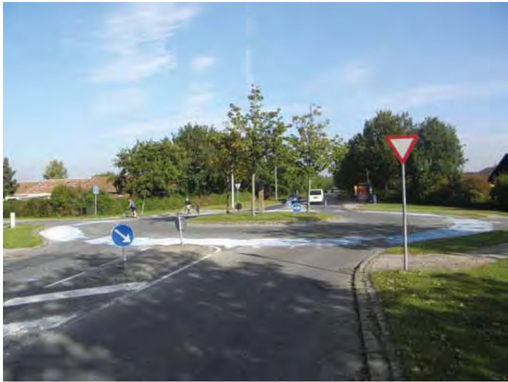
A large mini-roundabout; the cycle lane is probably not suitable.
