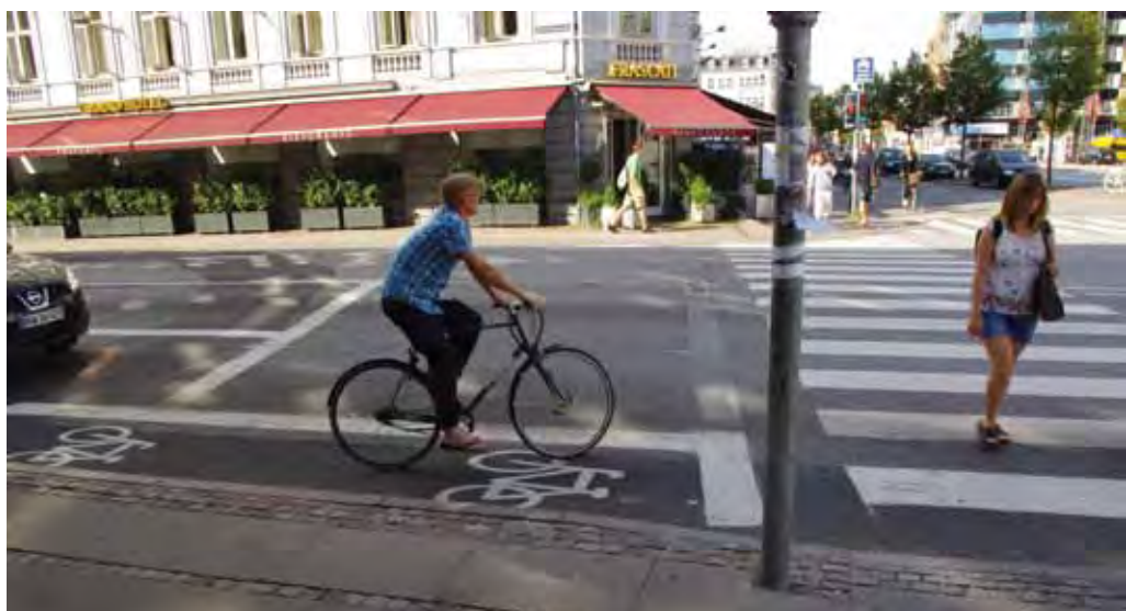
Narrowed bike lane leads into the intersection. Cyclists are visible and have their own area. Reventlowsgade, Copenhagen
