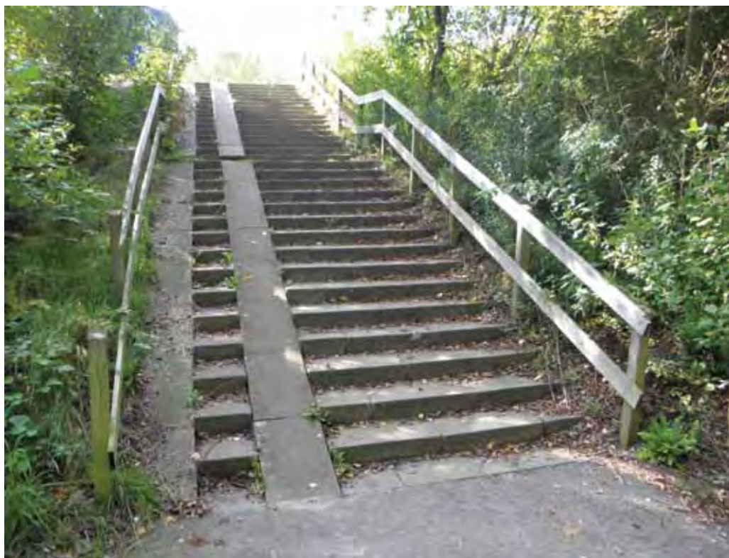
Combined bike and pram ramp.
