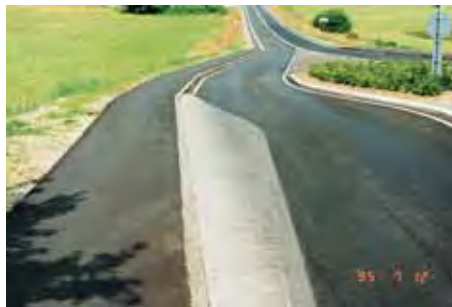
To prevent squeezing, cycle tracks or cycle lanes can be established by a median divider.
