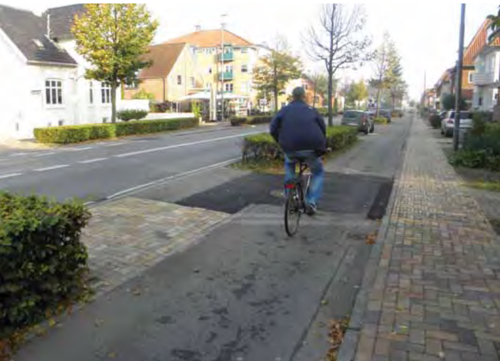
The pedestrian refuge between the cycle track and the carriageway enables pedestrians to cross the street more safely.
