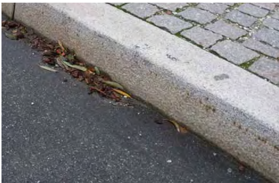
The traditional Danish cycle track with a curb provides excellent segregation between road user groups.
