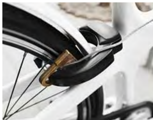
In Odense butterfly racks have been supplemented by a locking mechanism in the shape of a wire pulled up from the ground.
