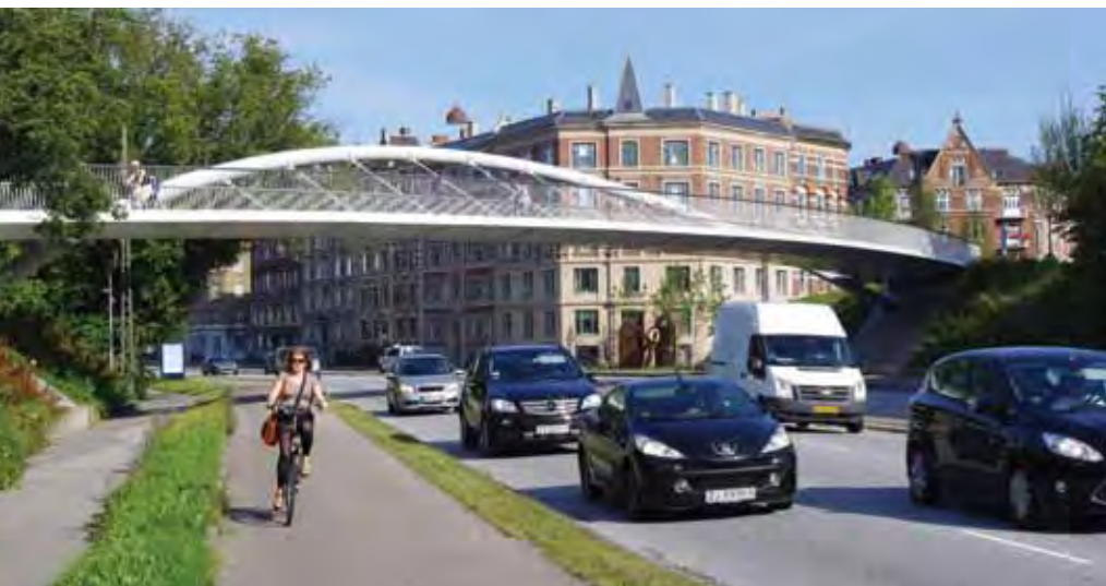
Åbuen. A bridge was the only feasible solution here as the alternative was a traffic signal which would significantly reduce motor vehicle capacity on this approach road. An underpass was not an option either since a stream runs under the road. The bridge links the municipalities of Copenhagen and Frederiksberg.
