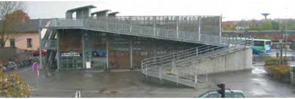
Bicycle parking garage with indoor and outdoor parking and bike shop, Næstved.
