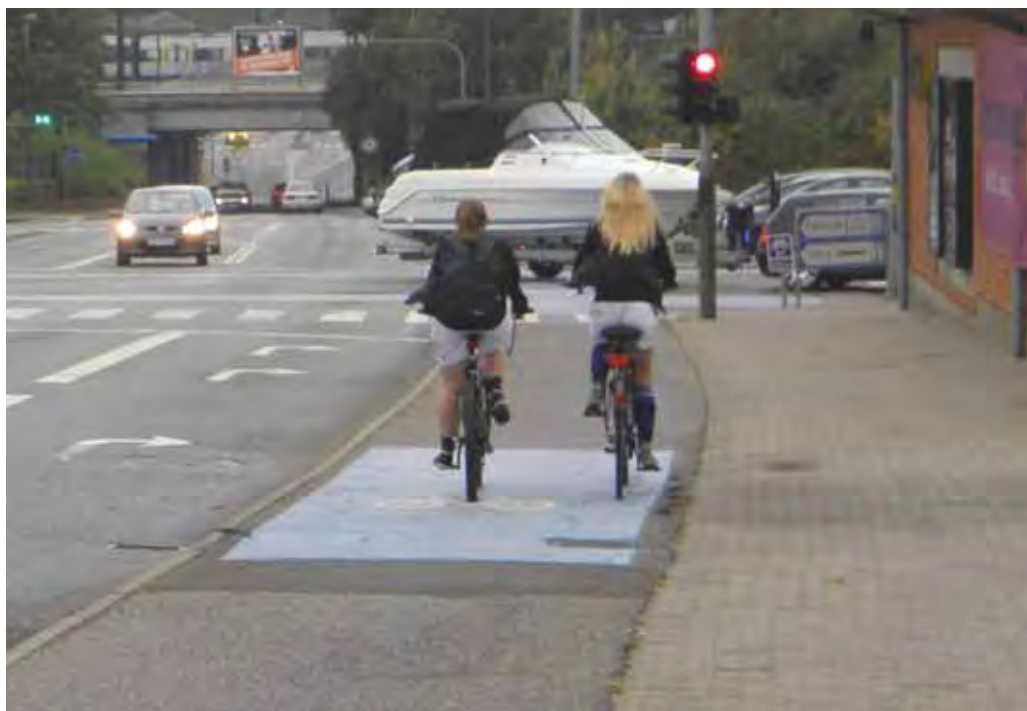
Blue cycle crossing on give-way controlled, continuous cycle track.
