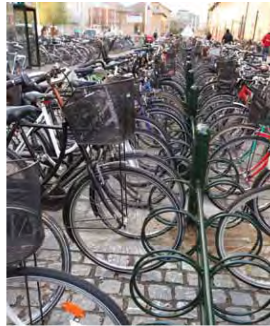
Two-sided butterfly rack, Frederiksberg. The stand is vertical and wedge shaped to fit different tire widths without damaging the tires.
