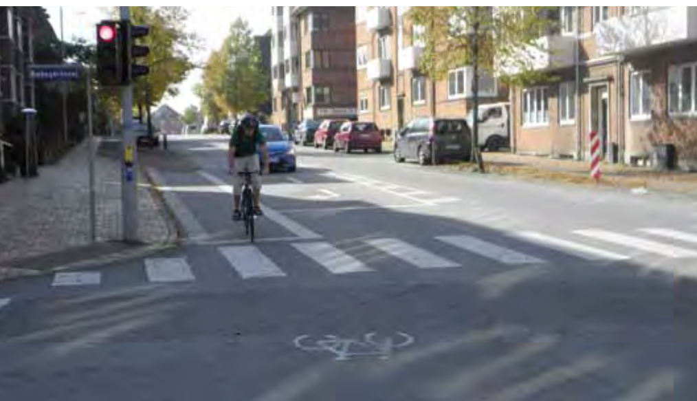
Shortened cycle track continued as a narrow cycle lane up to the stopline.
