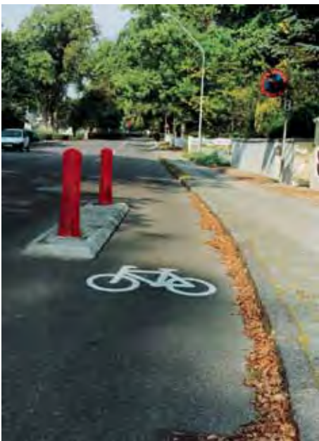
A good cycle gap is 1.4 m wide. If the gap is too narrow cyclists use the carriageway and if it's too wide, cars may use the gap.
