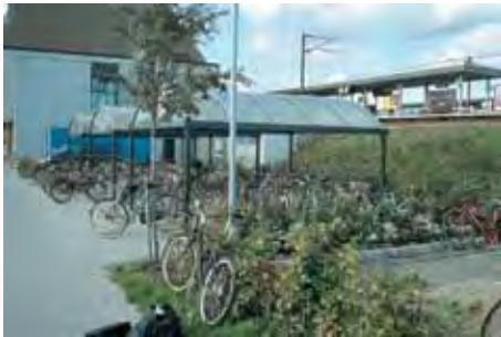
Covered bicycle parking facility at railway station
