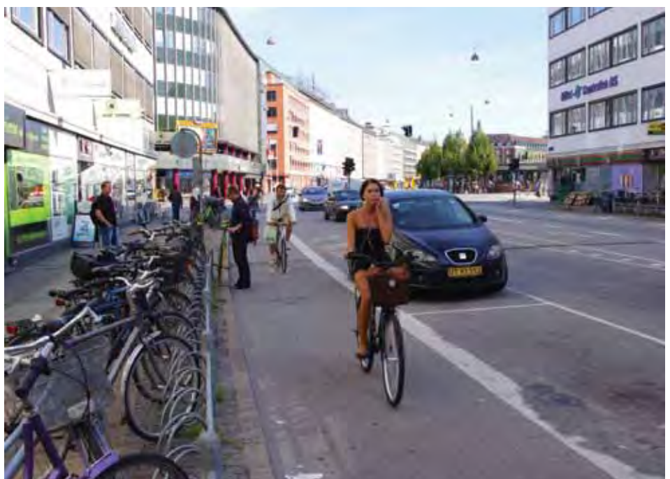
Car bays act as buffers protecting cyclists in the cycle lane. Farimagsgade, Copenhagen.
