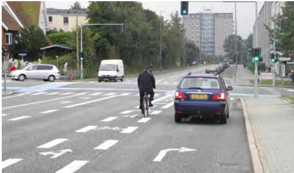
Cycle crossing between motor vehicles' right turn lane and lane for straight ahead traffic.
