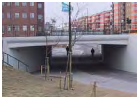
This Malmö cycle tunnel provides excellent visibility thereby enhancing cyclist's sense of security.
