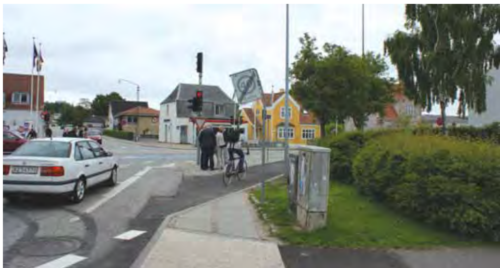
Shunt in Aalborg improves passability since cyclists needn't wait for the green signal before turning right.
