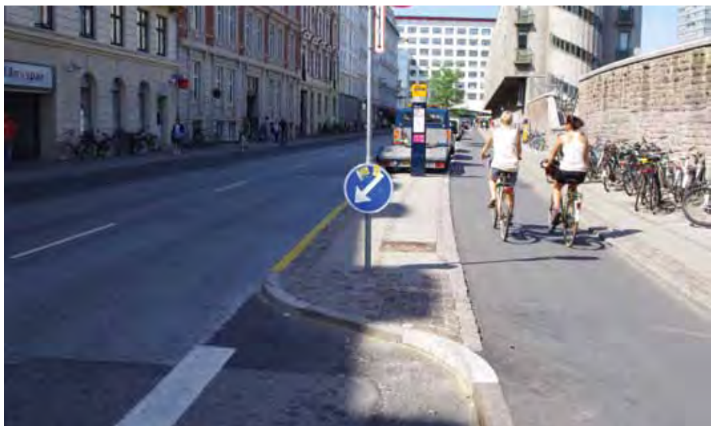
Bus nub (kerb extension) where the waiting area between the cycle track and the bus takes space from the cross profile. Car traffic – but not cycle traffic – has to wait while the bus stops at the bus stop.
